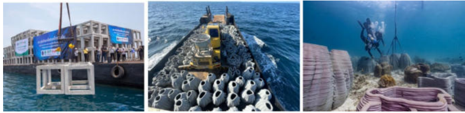
Fig. 1 The conventional artificial reefs installations in Thailand (Left; https://www.cpgroupglobal.com/en/newsroom/news/132/cp-group-launches-seacosystem-for-the-sustainable-thai-sea-integrating-support-from-all-sectors-for-the-conservation-of-thailand-s-sea-and-partners-with-the-department-of-fisheries-to-plant-1000-artificial-reefs , Center; https://esguniverse.com/content/251700/ , Right; https://www.dailynews.co.th/news/4158947/ )
