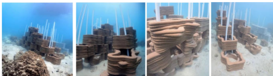
Fig. 15 Physical characteristics of the 3DMARs while installing (left to right), Image courtesy of Torpong Limlunjakorn
